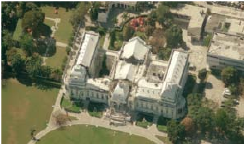
Figure 11. National Palace in Port-au-Prince after the earthquake and partial demolition, revealing the reinforced concrete frame infilled with rubble stone (© Pictometry).
