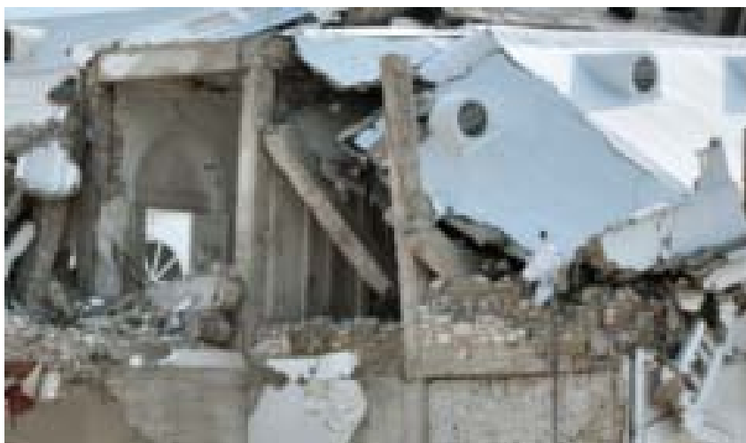
Figure 12. Detail view showing the reinforced concrete frame with round rock rubble stone infill of the 1916 structure exposed during the demolition of the ruins of the National Palace.
