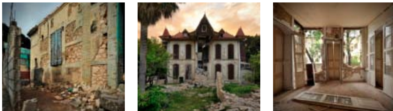
Figure 6. Brick and empanelled round-rock rubble stone construction, as is typically found in many of the Port-au-Prince "Gingerbread" Houses from the late 19th century, showing different levels of damage from onset, to collapse of the rubble panels. Center: The 2 1/2 story Villa Castel Fleuri Mansion was of rubble stone between brick piers and window surrounds, and only the staircase projection collapsed. The onset of inelastic deformation of the rubble stone panels is visible where the surface stucco has come off. Right: The Dufort House still standing on its brick piers after the collapse of the rubble stone panels. This house is now being restored by FOKAL. Many reinforced concrete buildings nearby collapsed.
