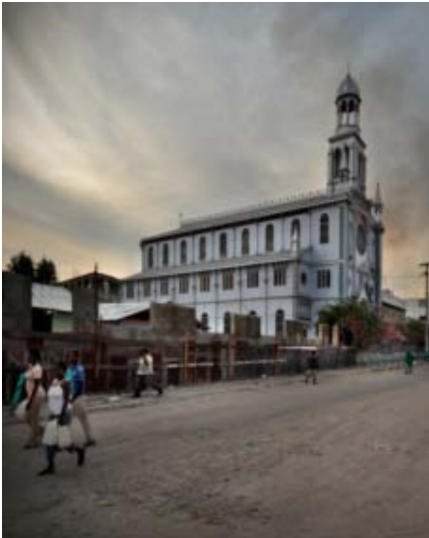
Figure 13. Saint Louis de Gonzague Chapel ca. 1890 in central Port-au-Prince showing external lightweight steel frame on masonry walls.
