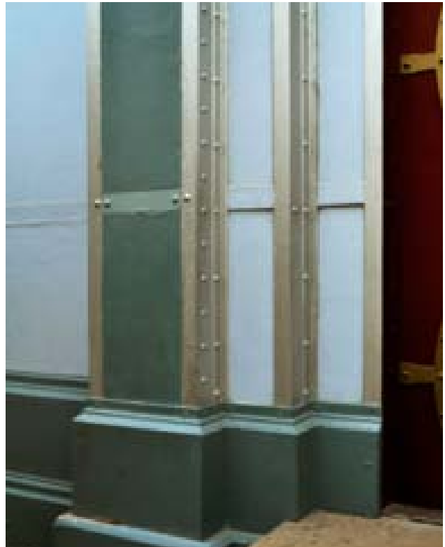
Figure 13. Saint Louis de Gonzague Chapel ca. 1890 in central Port-au-Prince showing external lightweight steel frame on masonry walls.
