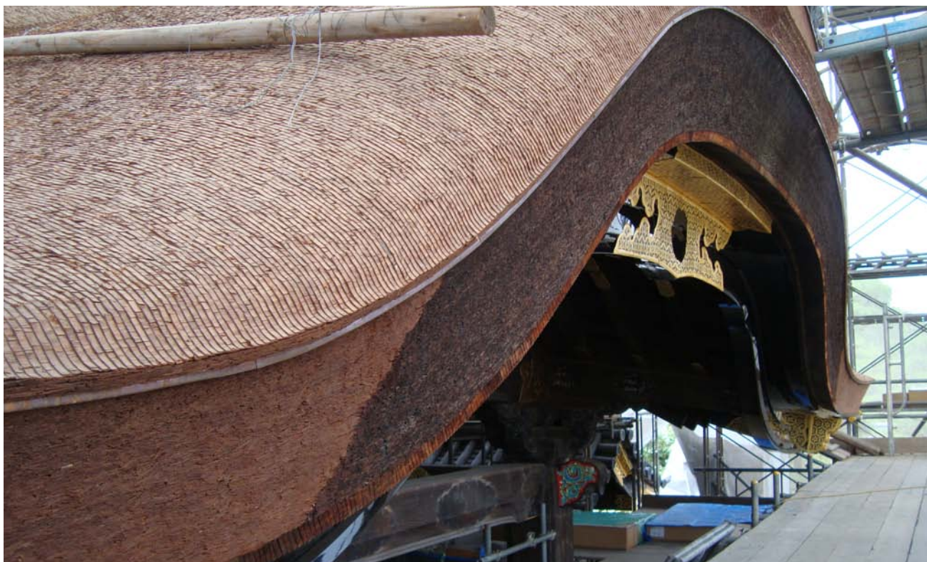
Kyoto. The restoration site of the Imperial gateway in Nijo Castle. June 25, 2013. Detail of the kara-hafu. The dark area is not restored. (2013 © Olimpia Niglio).
