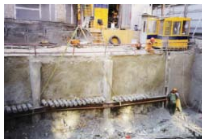
Fig. 9 Construction of the fore poles under the antiquities.
