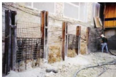
Fig. 9 Construction of the fore poles under the antiquities.
