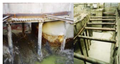
Fig. 11 Partial excavation and excavation to the final level.
