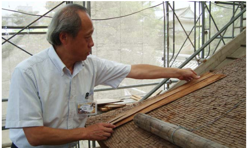
Kyoto. The restoration site of the Imperial gateway in Nijo Castle. June 25, 2013. The Architect Goto describes the restoration of roof with bark of the cypress. (2013 © Olimpia Niglio).
