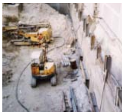
Fig. 8 The “Berlin” type of wall used for the temporary support of the excavation slopes.
