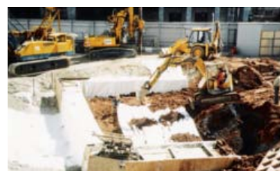
Fig. 6 Protection of the antiquities before earth filling.
