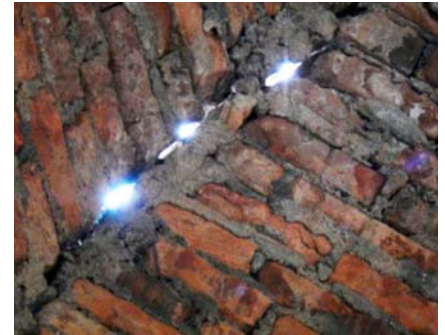
Figure 11. Fissures on caskets of the dome of the temple of Santa Lucía (Source: by the authors).
