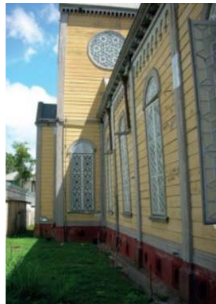
Figure 15. Rigid rotation of the wall of the side nave (Tampone, Atlas, 2016, cit.).
