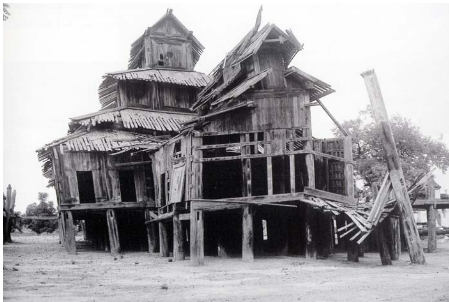
Figure 14. Rigid rotation of one of the bodies of a timber building in Myanmar (from Tampone, Atlas, 2016, cit.).
