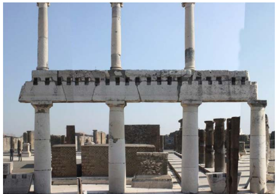
Figure 1. The forum of Pompeii: (a) Aerial view of the southern part of the Forum showing the colonnade under investigation inside the circle; (b) Two storeys colonnade with multi-drum columns and multi-blocks segmented trabeations.
