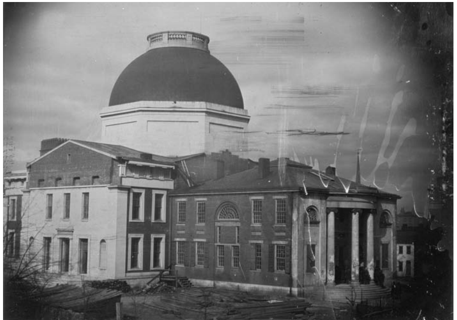
FIGURE 4. Southeast view of the courthouse in 1851, just before demolition of the previous courthouse and construction of the east wing. The first courthouse completed in 1828 is visible at right, with the south transept and west wing visible at left. Source: Half plate daguerreotype by Thomas Easterly taken in 1851. Missouri History Museum collection, reference n17030.
