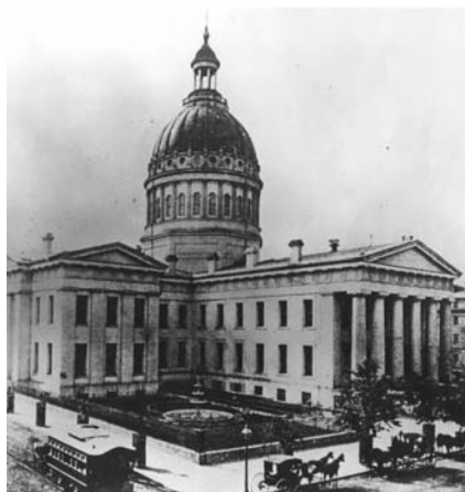
FIGURE 19. The southeast courtyard, 1866. This 1866 view of the southeast courtyard illustrates the southeast courtyard, including the fountain surrounded by a wrought iron fence, perimeter fence and wall, walk leading to the south wing areaway, and street trees set within the sidewalks edging the city streets. Source: JNEM Archive. "The view from the southeast in 1866, shortly after completion of the dome.
