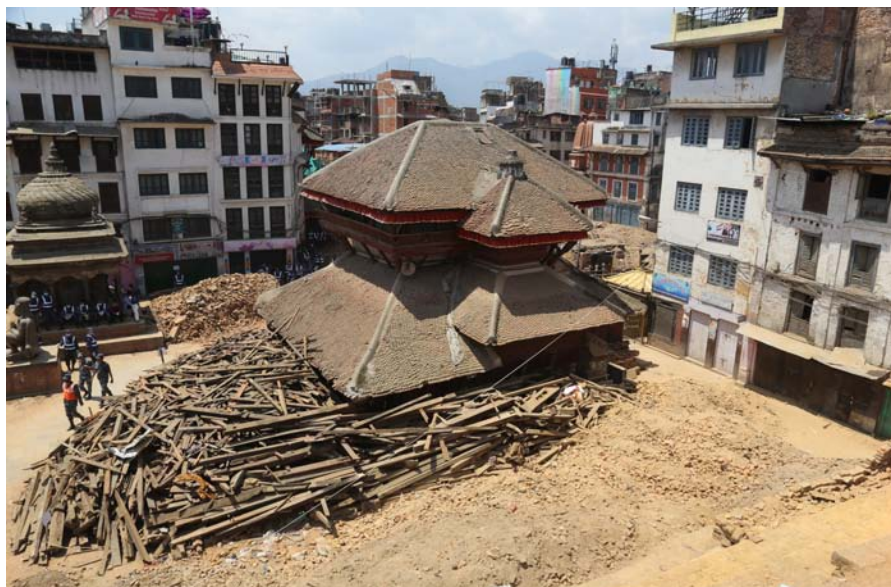
Nepal Earthquake (photo: Dinçşahin, Umut, GEA Conference 12.12. 2015).
