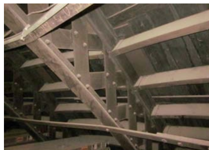
FIGURE 16. The dome ribs are lattice work, radially laid members constructed of structural T-shapes for the inner and outer flanges, with plates riveted to the stems of the T-sections and at the intersection of the plates. The 2x6 wood purlins are fastened to the outer T-section with metal joist hangers to provide a nailable surface for the wood plank sheathing below the sheet metal copper roofing.
