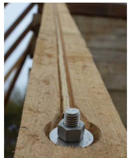
Figure 6 Synthetic rope used for flexural strengthening of the first common rafters. A stainless steel bolt anchors the end-loop, and the rope is recessed in a small channel along the top of the timber (photo by Sarah Marie Jackson).
