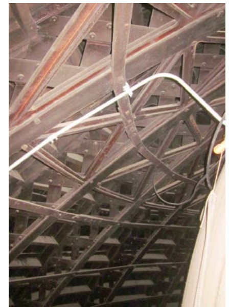
FIGURE 17. View of the dome ribs and radial straps. The straps are located only in the lower portion of the dome, where the outward thrust would be greatest.
