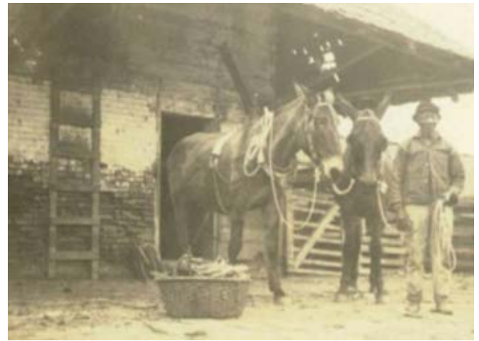
Figure 2 Documentary evidence for the lack of columns at the roof edge: Left, as remembered by artist Clementine Hunter, and right, as seen in the earliest known photos.
