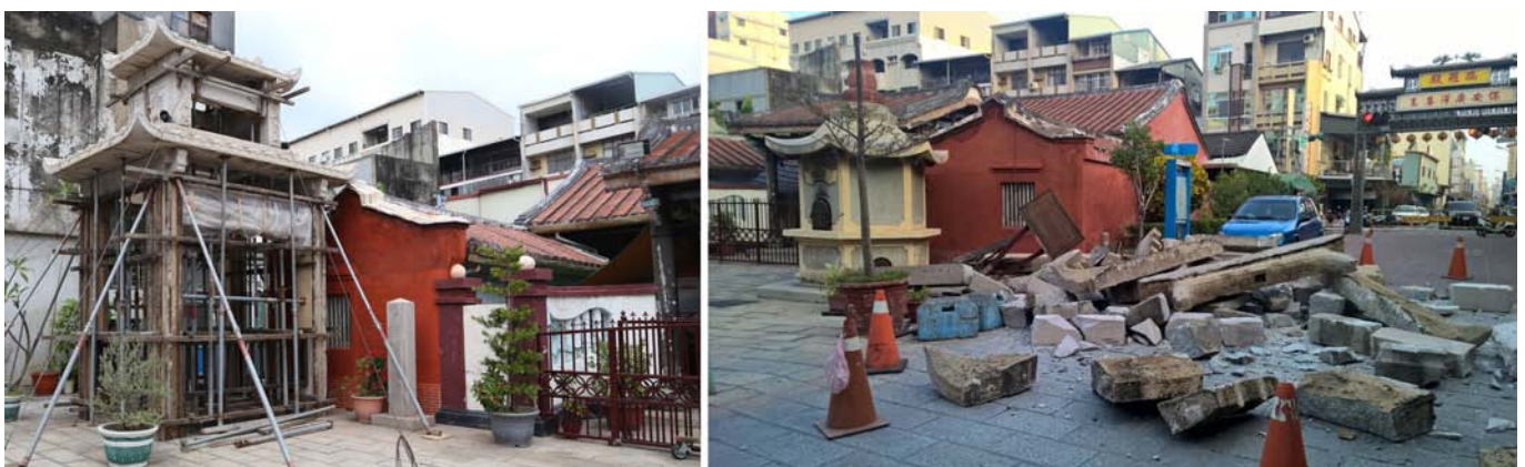
Figure 5: Wind God Temple. Left: Drum Tower (Photo: http://www.fingermedia.tw/ ). Right: Collapsed Bell Tower. The furnace is also damaged. (Photo: Tainan Municipal Administration of Cultural Heritage).
