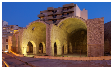
Figure 1: Photo of one of the barrel vault structures of the Venetian dockyards at Heraklion Crete (Greece), by C messier, Wikimedia Commons, licensed under CC BY-SA 4.0
