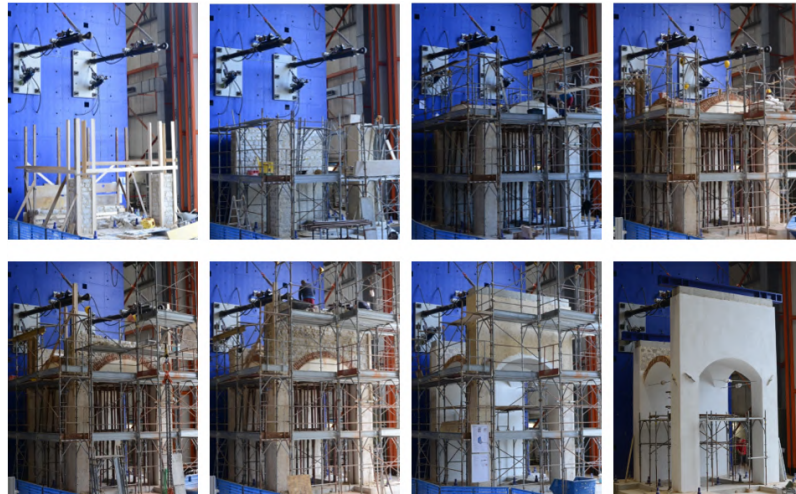
Figure 2: Construction sequence of the specimen
