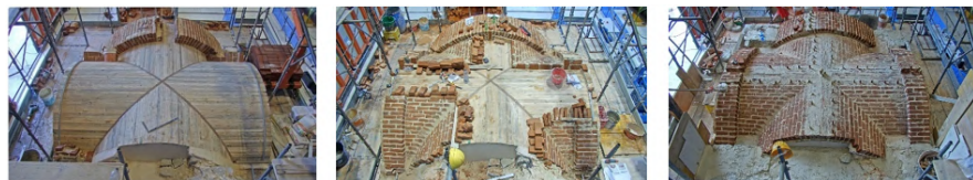
Figure 3: Construction sequence of the vault and arches
