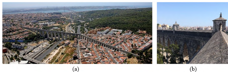
Figure 1: (a) Águas Livres Aqueduct. Neighbourhoods Serafina on the right; Campolide on the left. (b) Canal gallery, lanterns and lateral walkways
