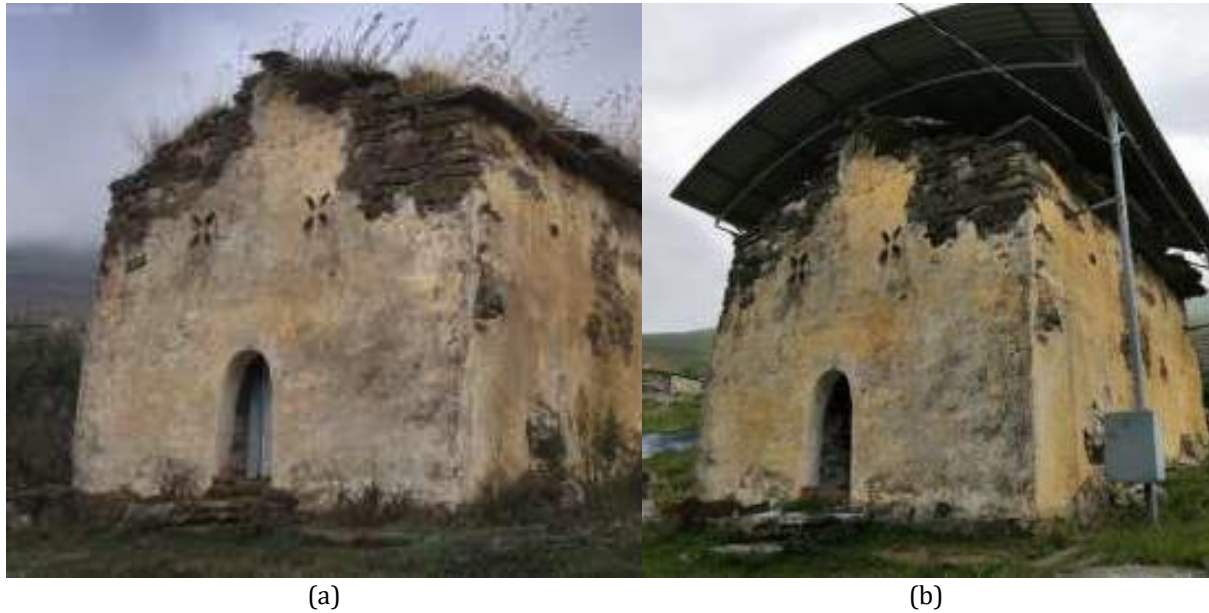
Figure 9: (a) The Faraskatta church before conservation, (b) Conservation roof installed in the 1990s
