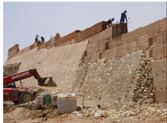
(a) (b) Figure 6: (a) Aerial view of the Kasbah Agadir Oufella rehabilitation (Salima Naji) (b) Wall construction and reinforcement technique, Kasbah Agadir Oufella (Salima)
