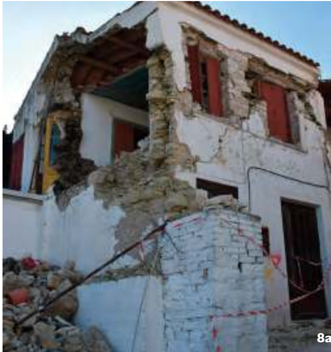
Figures 8. The effect of separation of the leaves of masonry: 8a. In-plane shear and partial out-of-plane collapse of a three-leaf wall and 8b. Out-of-plane collapse of the central region of a wall.
