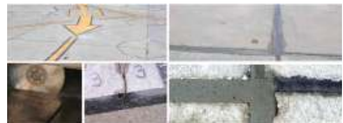
Figures 19. The repair flexible joint made of polyurethane PM, resistant to environmental and chemical factors acting on the joints at the cracked concrete airfield slab in the Cracow-Balice Airport.
