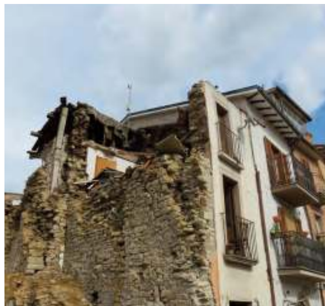
Figure 20. The out-of-plane bending of multi-leaf masonry elements may lead to separation among the leaves and to out-of-plane collapse of the outer leaf.
