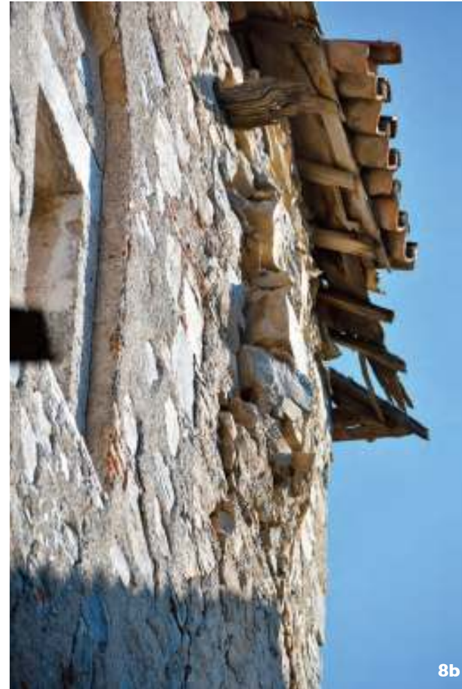
Figures 8. The effect of separation of the leaves of masonry: 8a. In-plane shear and partial out-of-plane collapse of a three-leaf wall and 8b. Out-of-plane collapse of the central region of a wall.
