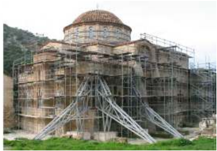
Figure 4. Raking shores installed in the NE corner [5] © Hellenic Ministry of Culture.
