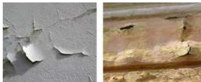
Figure 8. Examples of surface layer blossoming damage.
