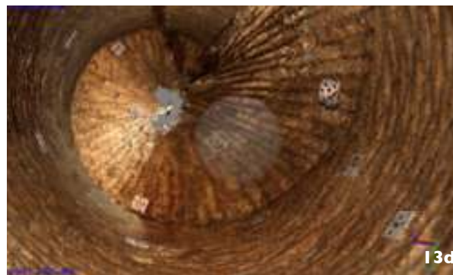
Figures 13. Close range photogrammetry of the minaret, cloud point samples: 13a. outer side, 13b. close-up outer side, 13c. and 13d. inner side.
