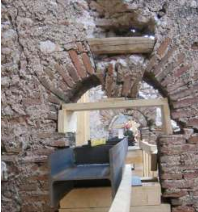
Figures 5. Hinges on the arch.
