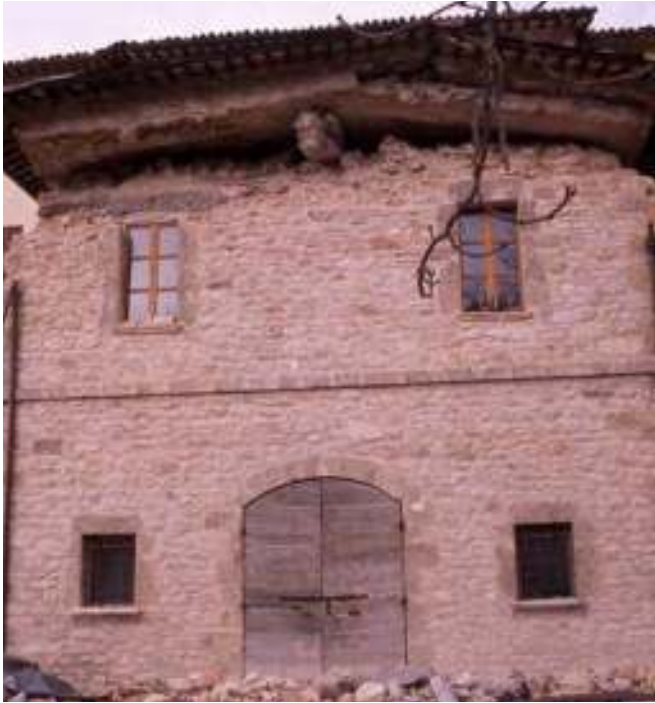
Figure 6. Hammering of RC roof.
