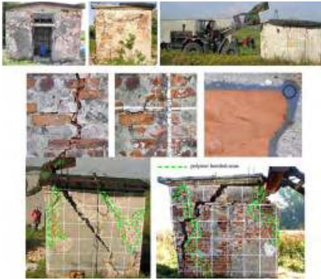
Figures 13. Dynamic in situ tests up to failure on small cracked masonry building, repaired by flexible joints made of polyurethane PM.
