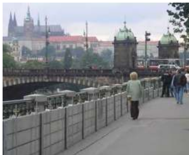
Figure 12. Example of temporary protecting wall.
