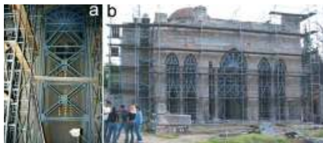
Figures 5a. Vertical steel props in the interior and 5b. in the exonarthex [5] © Hellenic Ministry of Culture.
