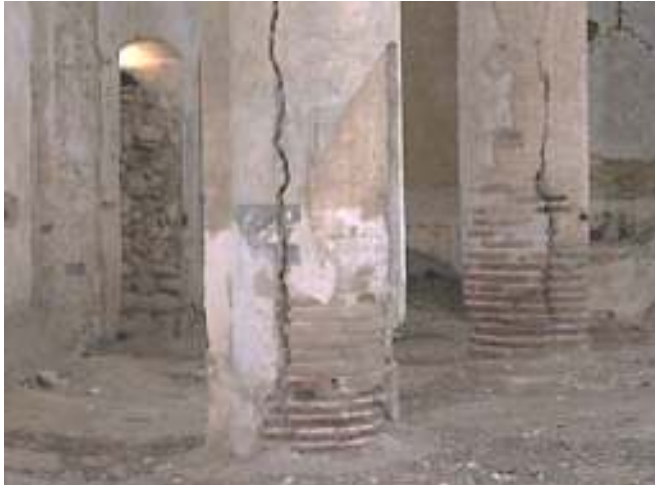
Figures 1a. Vertical cracks; 1b. Loss of the material.
