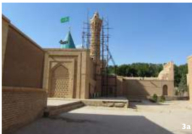
Figures 3. General photos and images showing different parts of the minaret: 3a. location within the complex, 3b. eastern side, 3c. eastern side, as photographed few decades ago, 3d. lower portion of western side, photographed few decades ago, 3e. entrance to the minaret (at its eastern side, 3f. lower side of the spiral staircase connected to the minaret shell, 3g. upper side of the spiral staircase.
