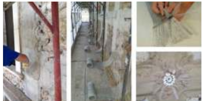
Figures 24. Composite strengthening of an historical building in L'Aquila (Italy), courtesy of Kerakoll.
