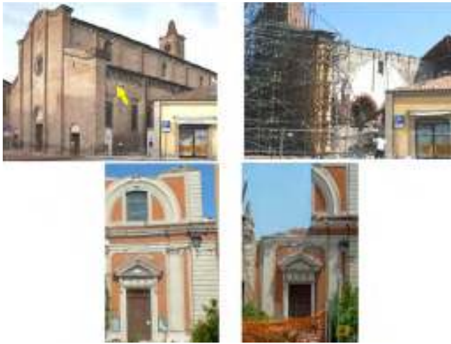
Figures 2. Damages of the church of San Francesco in Mirandola (top) and of the church of D.O.M. in San Felice sul Panaro (bottom), caused by the first shock and the aftershocks [8].
