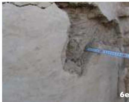
Figures 6a. Diagonal crack at the south-western side (filled with mortar), 6b. diagonal crack at the south-western side, photographed few decades ago, 6c. diagonal crack at the south-eastern side and vertical crack at the southern side, 6d. and 6e. external side of the hole at the northern side filled with mortar, 6f. internal side of the hole at the northern side filled with bricks, 6g. holes at the north-western side, 6h. and 6i. cracks inside the minaret, 6j. external layer on the main shell of the minaret near the apex.
