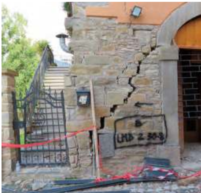
Figures 16. Walls subjected to large lateral displacements.
