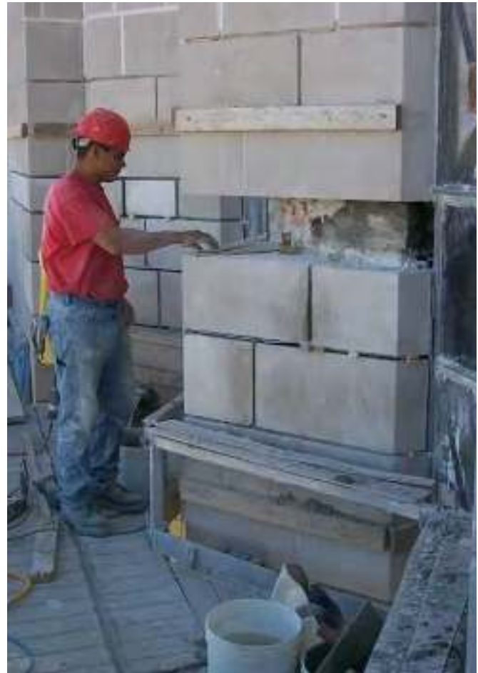
Figure 3. As part of the therapy on the 121 meter tall Nebraska State Capitol, USA the limestone units were selectively removed to expose the steel support structure beneath so that the corrosion could be removed, the steel painted, and flashed prior to reinstallation of the limestone.
