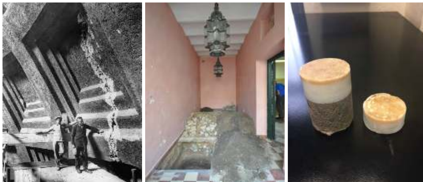
Figure 7. Prof. Giacomo Boni, famed Italian archaeologist, inspects a crack in the concrete vaulting of the dome of the Pantheon during restoration in 1925. Figure 8. Sondage at the Tangier American Legation Museum Pavilion Arabe in Morocco (early 20 th Century) to determine the makeup of the foundations. Figure 9. Removal of cores through the marble floor of the Oklahoma State Capitol (1914-1918) to determine the depth of the marble staining.
