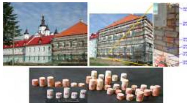
Figure 29 Micro-cores from bricks from South-East part of the Supraśl Monastery (Poland).
