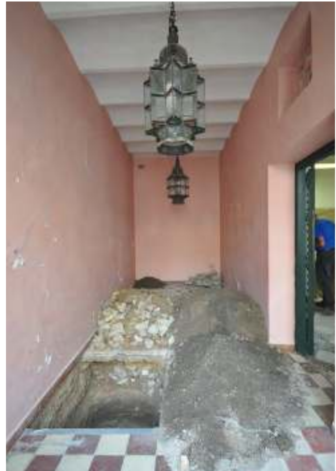
Figure 2. At the Tangier American Legation Museum in Morocco a sondage was required to expose the foundation systems as part of diagnosing issues with building settlement.
