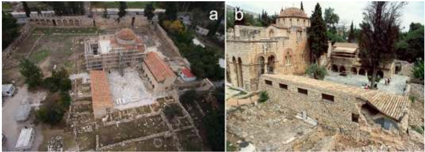
Figures 1a. The Monastery from S-W during restoration and 1b. after the earthquake [8] © Hellenic Ministry of Culture.
