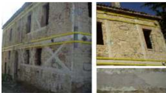
Figures 25. Seismic retrofitting of a damaged masonry building in San Marino, courtesy of Kimia.
