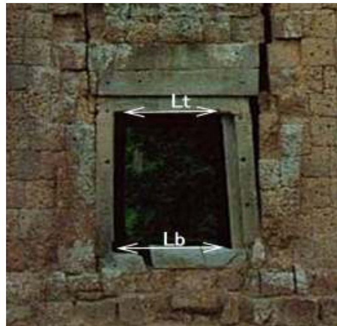
Figure 9. Open window of the west side of NI Tower.
