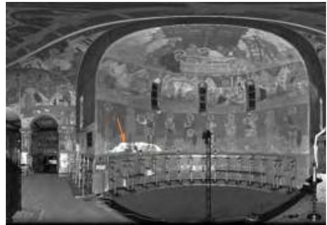
Figure 19. Salt efflorescence recorded by laser scanning in orthodox church in Chevetogne, Belgium (scan author).
