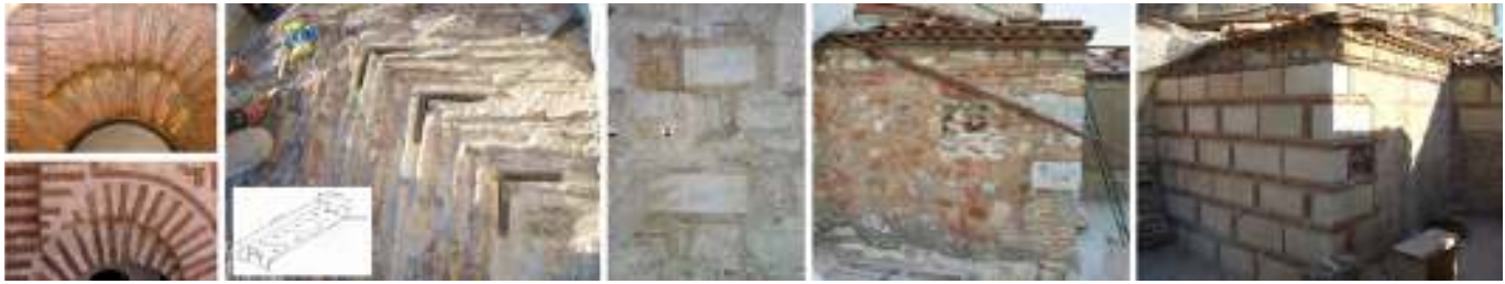
Figure 25. First phase structural restoration interventions (removal of 1960's cement re-pointing mortars, stitching of cracks with titanium plates or stones and local reconstruction to correct past alterations) adapted from [9] © Hellenic Ministry of Culture.
