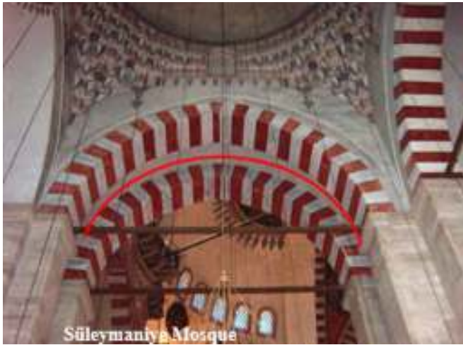
Figure 10. Seismic joints in Süleymaniye Mosque and Çifte Hamman.
