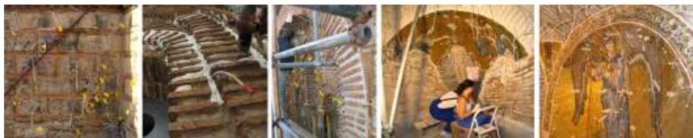
Figure 27. Preparation for grouting of masonry, bearing old mortars and of mural mosaics adapted from [9] © Hellenic Ministry of Culture.
