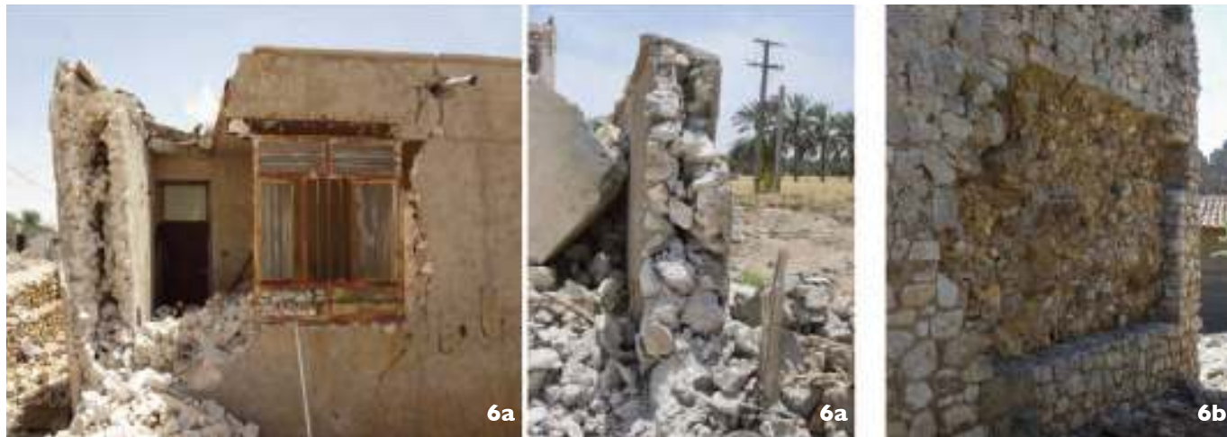
Figures 6. Three-leaf masonries in: 6a. Iran [6] and 6b. Greece.
