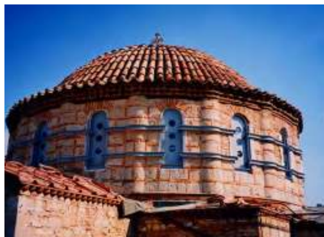
Figure 6. Dome's windows bracing [5] © Hellenic Ministry of Culture.
