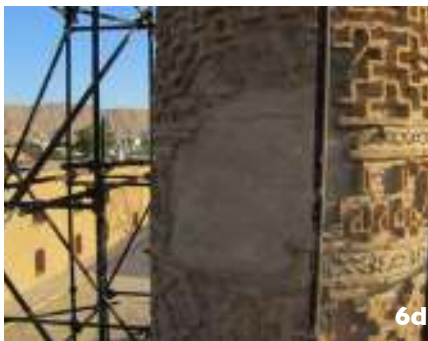
Figures 6a. Diagonal crack at the south-western side (filled with mortar), 6b. diagonal crack at the south-western side, photographed few decades ago, 6c. diagonal crack at the south-eastern side and vertical crack at the southern side, 6d. and 6e. external side of the hole at the northern side filled with mortar, 6f. internal side of the hole at the northern side filled with bricks, 6g. holes at the north-western side, 6h. and 6i. cracks inside the minaret, 6j. external layer on the main shell of the minaret near the apex.
