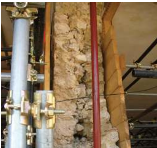
Figure 20. The out-of-plane bending of multi-leaf masonry elements may lead to separation among the leaves and to out-of-plane collapse of the outer leaf.
