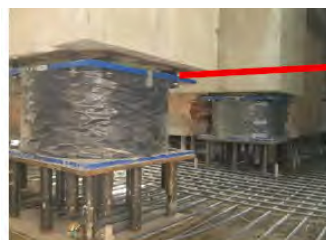
a) Rubber bearings installed on steel tables with anchor bolts, which remain embedded into the inferior carrying frame
