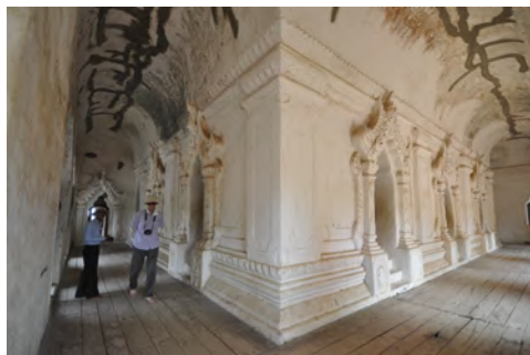
Figure 5: View of the lower gallery from the southwest showing the cracks along the apex of the vaults (S. Kelley photo).
