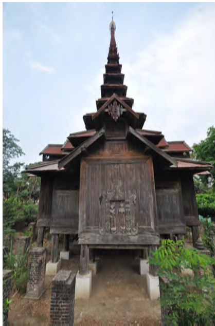
Figure 3: The monastery of Thin-gaza has its teak posts replaced above grade with square concrete piers due to rot and termite damage (S. Kelley photo).
