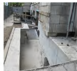
c) The isolation gap for which a concrete cover was made to protect people and objects from falling into the gap
