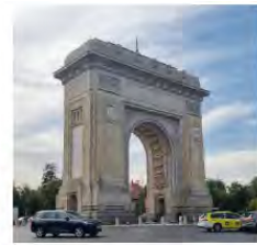
c) Arch of triumph (Bucharest) isolated with rubber bearings + viscous dampers
