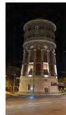
e) Fire Tower (Bucharest) isolated with rubber bearings + viscous dampers
