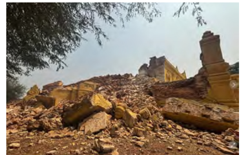
Figure 6: The collapse of the Maha Aungmye Bonzan Kyaung following the earthquake (photo from the Associated Press)
