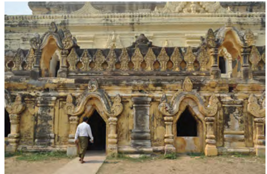
Figure 4: View of the Maha Aungmye Bonzan Kyaung from the south revealing the intricate ornamentation rendered in stucco over brick masonry (S. Kelley photo).
