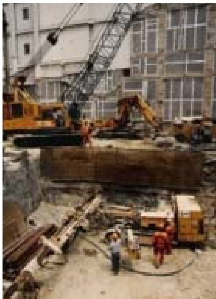
Fig. 19. Construction of the fore poles under the antiquities.
