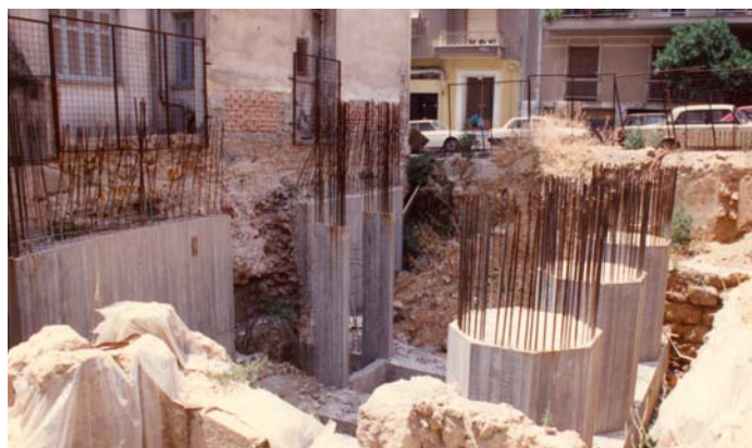
Fig. 45. Foundation of the 18 Erechtheiou Str. building; Figs. 46a, 46b. The foundation and the columns of the basement of the 18 Erechtheiou Str. building.
