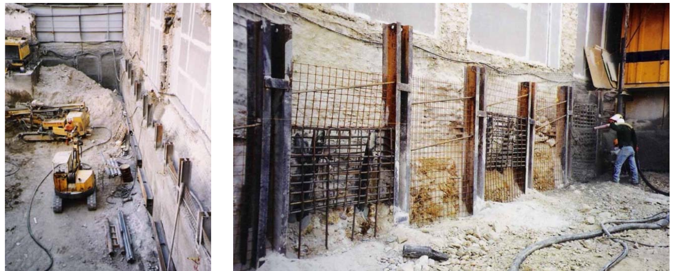
Fig. 18. The "Berlin" type of wall used for the temporary support of the excavation slopes.
