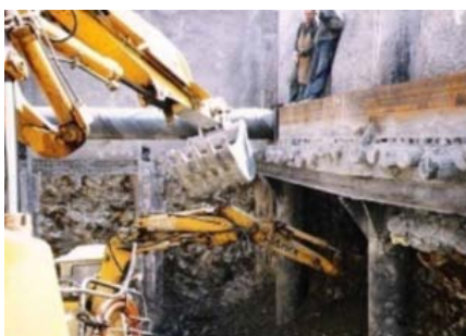
Fig. 21. Excavation under the antiquities. Temporary support with steel frames.
