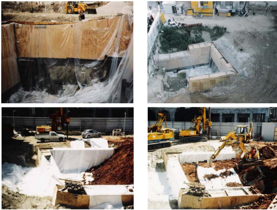
Fig. 16. Protection of the antiquities before earth filling.
