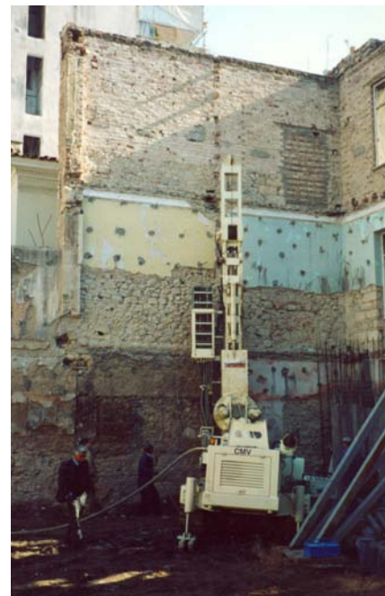
Fig. 35. Construction of micro piles at the Benaki Islamic Art Museum.
