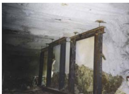
Fig. 21. Excavation under the antiquities. Temporary support with steel frames.
