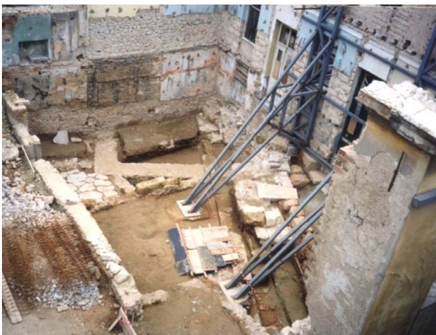
Fig. 32. Buttrressing of the facades of the twostorey building of the Islamic Art Museum.
