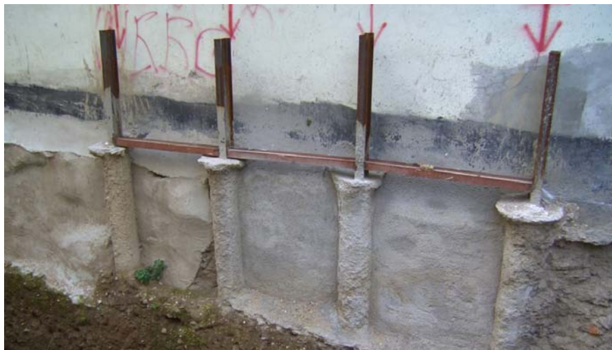
Fig. 29. Detail of the temporary support of a neighbouring structure at the Cherefontos cite.
