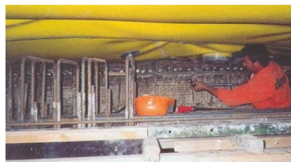
Figs. 23 and 24. Details of the preparations for concreting the slabs under the antiquities.
