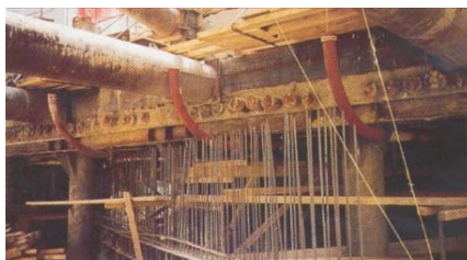
Figs. 23 and 24. Details of the preparations for concreting the slabs under the antiquities.
