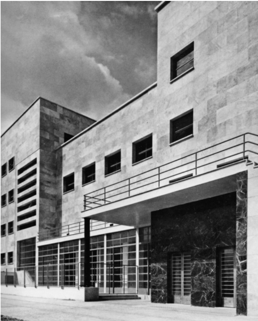
The swimming pools façade, 1937. The cladding was realised using 2 cm thin Carrara marble panels (Archivio Centrale dello Stato, Fondo Gaetano Minnucci, busta 147, fascicolo 260).
