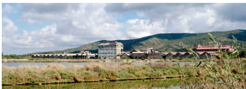
The artificial canal in front of the plant (2013 © Micco F. I.).
