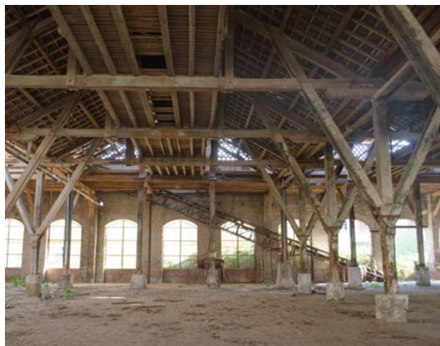
The Superphosphate warehouses: interiors (2013 © Micco F. I.).
