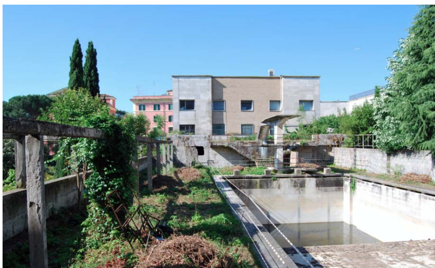
The outdoor swimming pool, 2014. The whole area is infested by weeds; the flooring is almost completely lost; the marble covering of the basin is heavily damaged by the presence of stagnant water.
