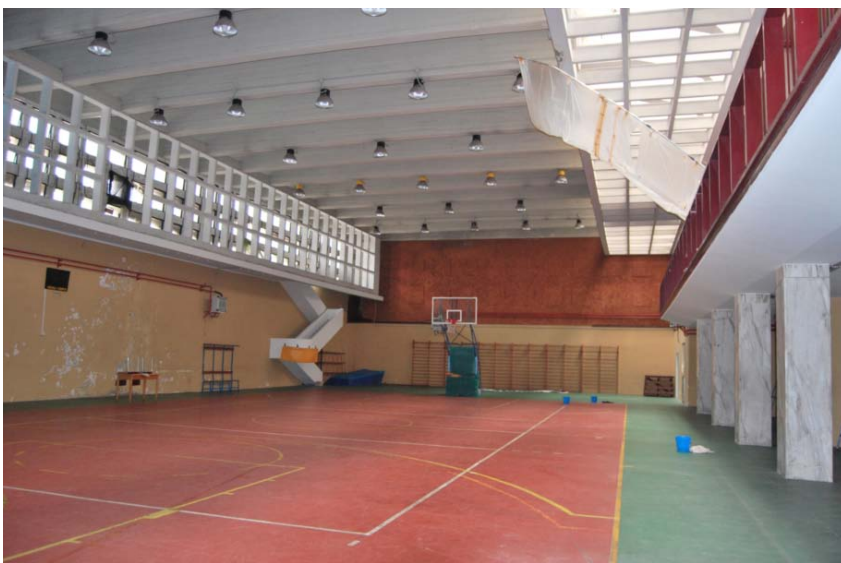
The gym before the last restoration works, occurred between 2013 and 2014.
