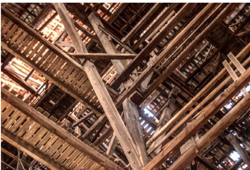
A detail of the wooden carpentry (2013 © Micco F. I.).
