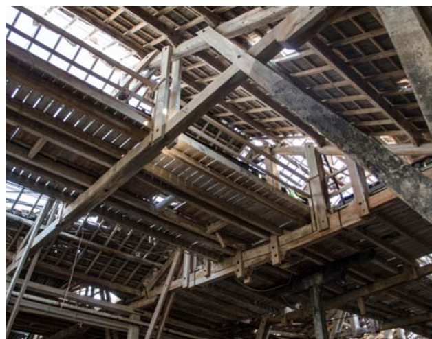
The Superphosphate warehouses: footbridge detail (2013 © Micco F. I.).
