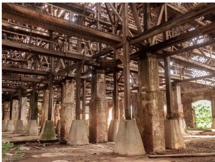
The lead-chambers area (2013 © Micco F. I.).
