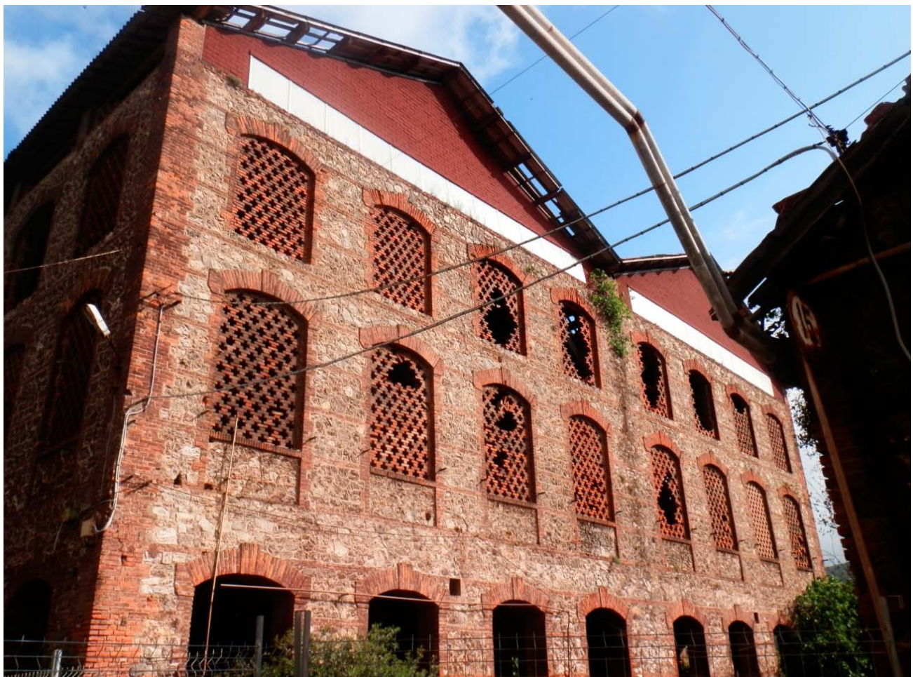
The masonry façade (2013 © Micco F. I.).
