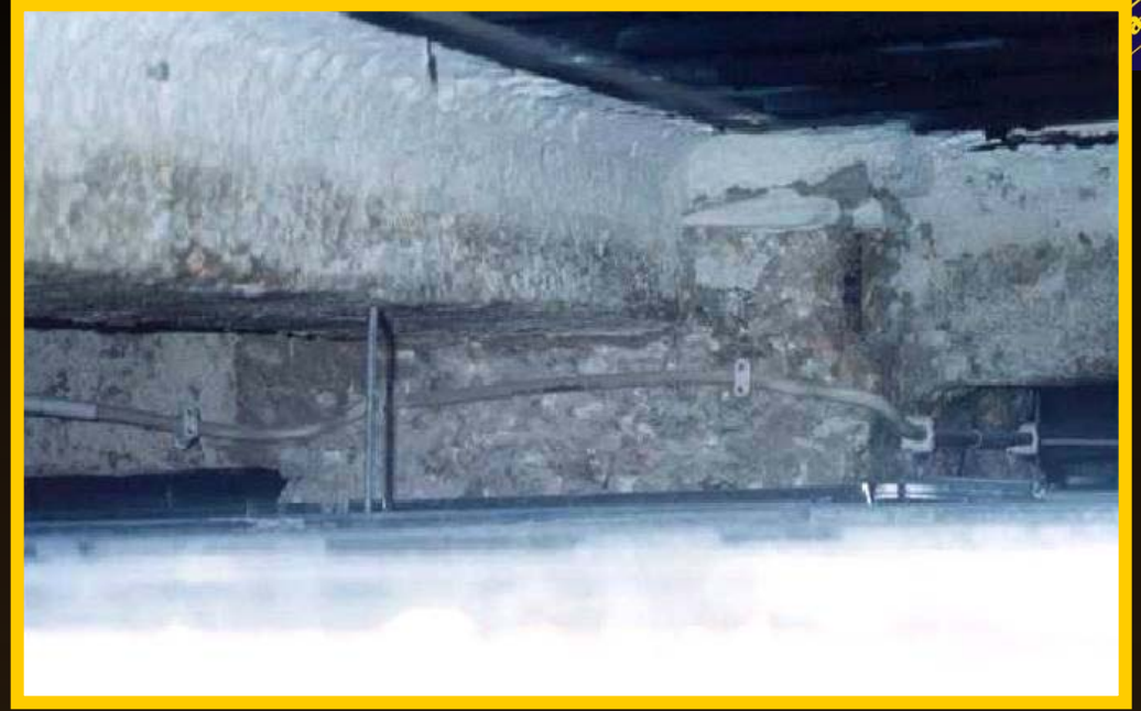
Execution of new RC slabs at ground level.
