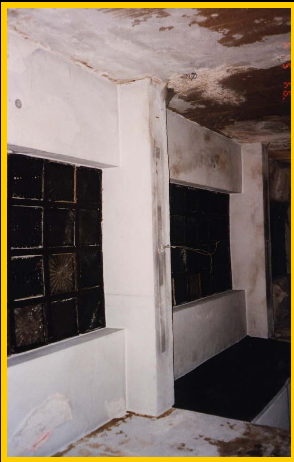
Alteration of the structural system with replacement of masonry components by reinforced concrete.
